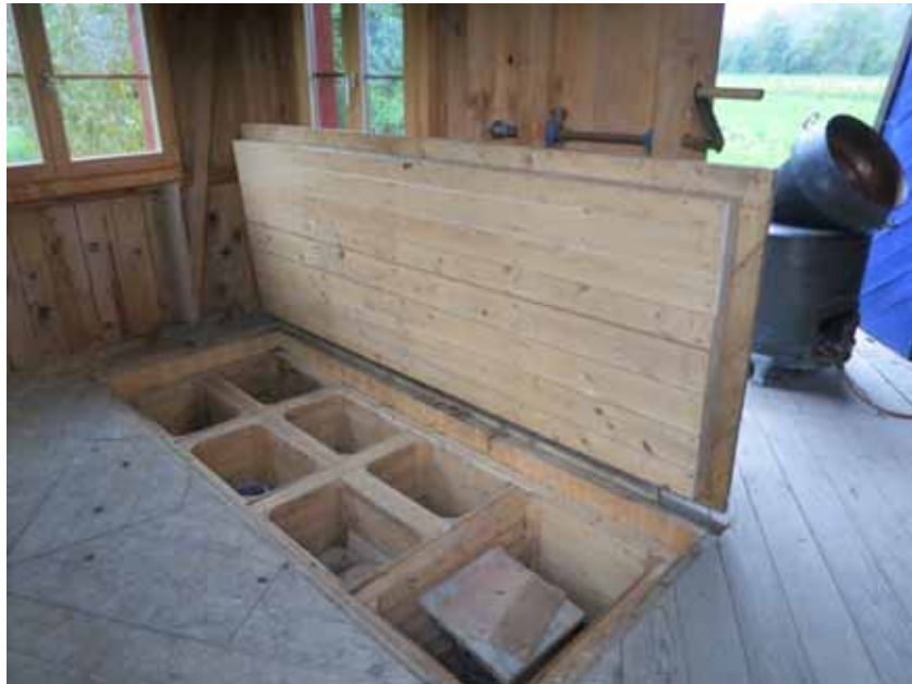
Picture 3-8: The preparation storage box: sunk into the floor of the preparation house
